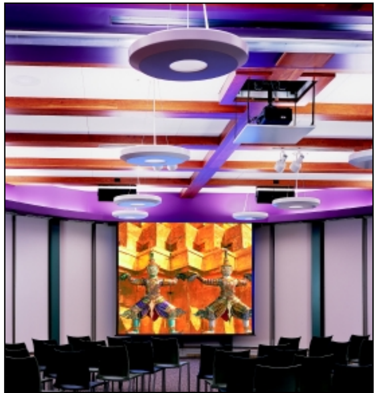
Photo: Carmel Clay Public Library Program Room, Carmel, IN. Installation includes ELECTRAMOUNT projector lift and FLEXSHADE DUAL ROLLER SYSTEM for glare control and room darkening.
